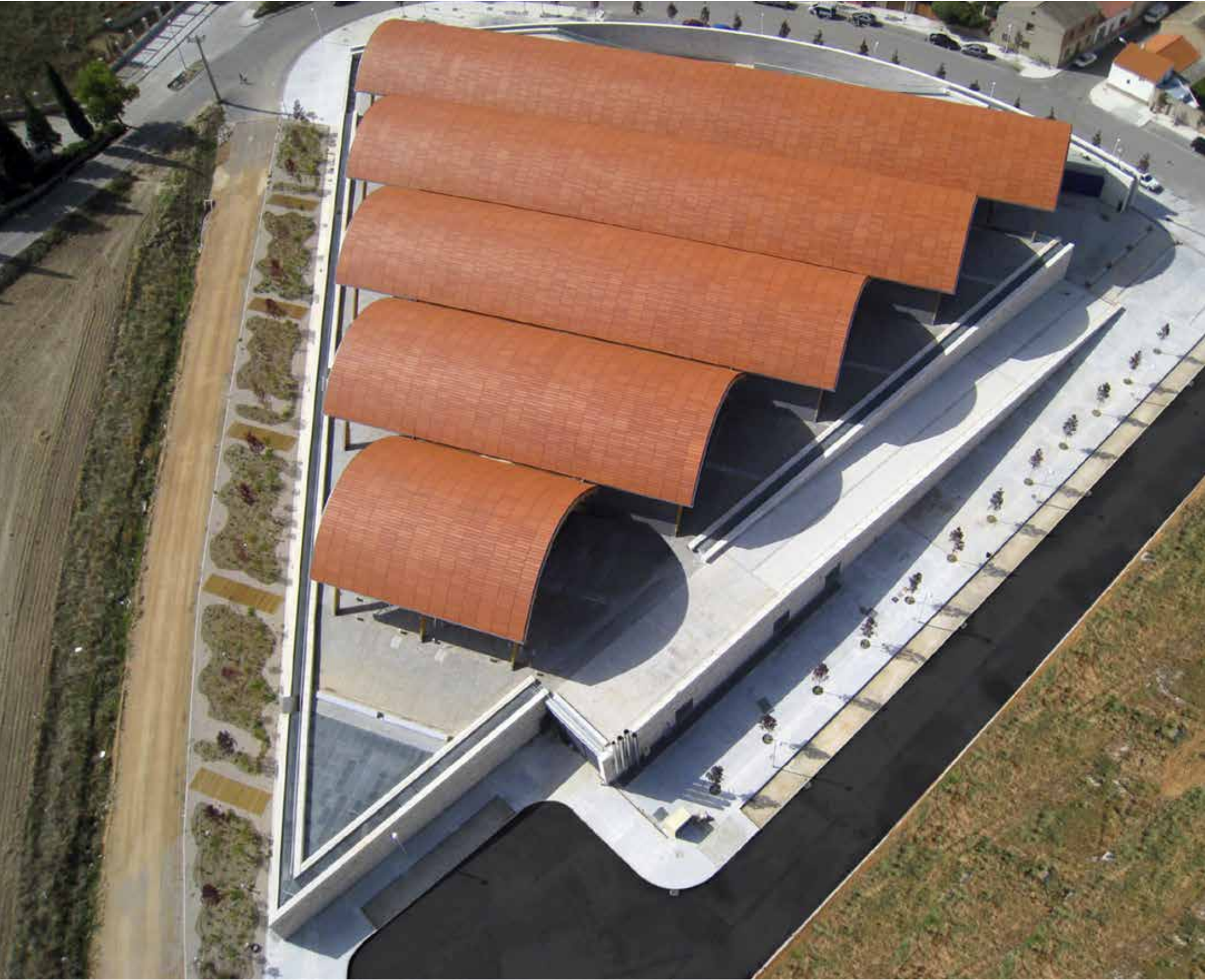
Aerial view of the roof | Photographer Bodegas Protos | Copyright holder Bodegas Protos
