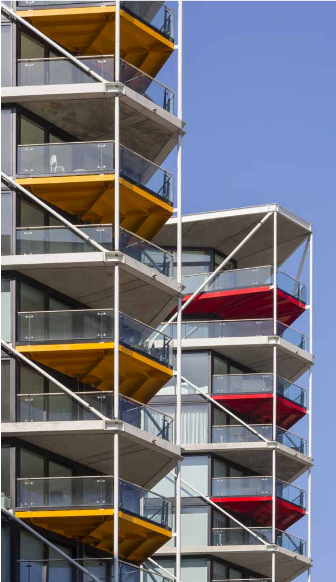
Paul Raftery | Battersea, London, Riverlight, Rogers Stirk Harbour and Partners, architecture, atrium, iconic, modern | Mid-levels are represented as concrete floors expressed every two storeys, with intermediate floors expressed as lightweight steel balconies
