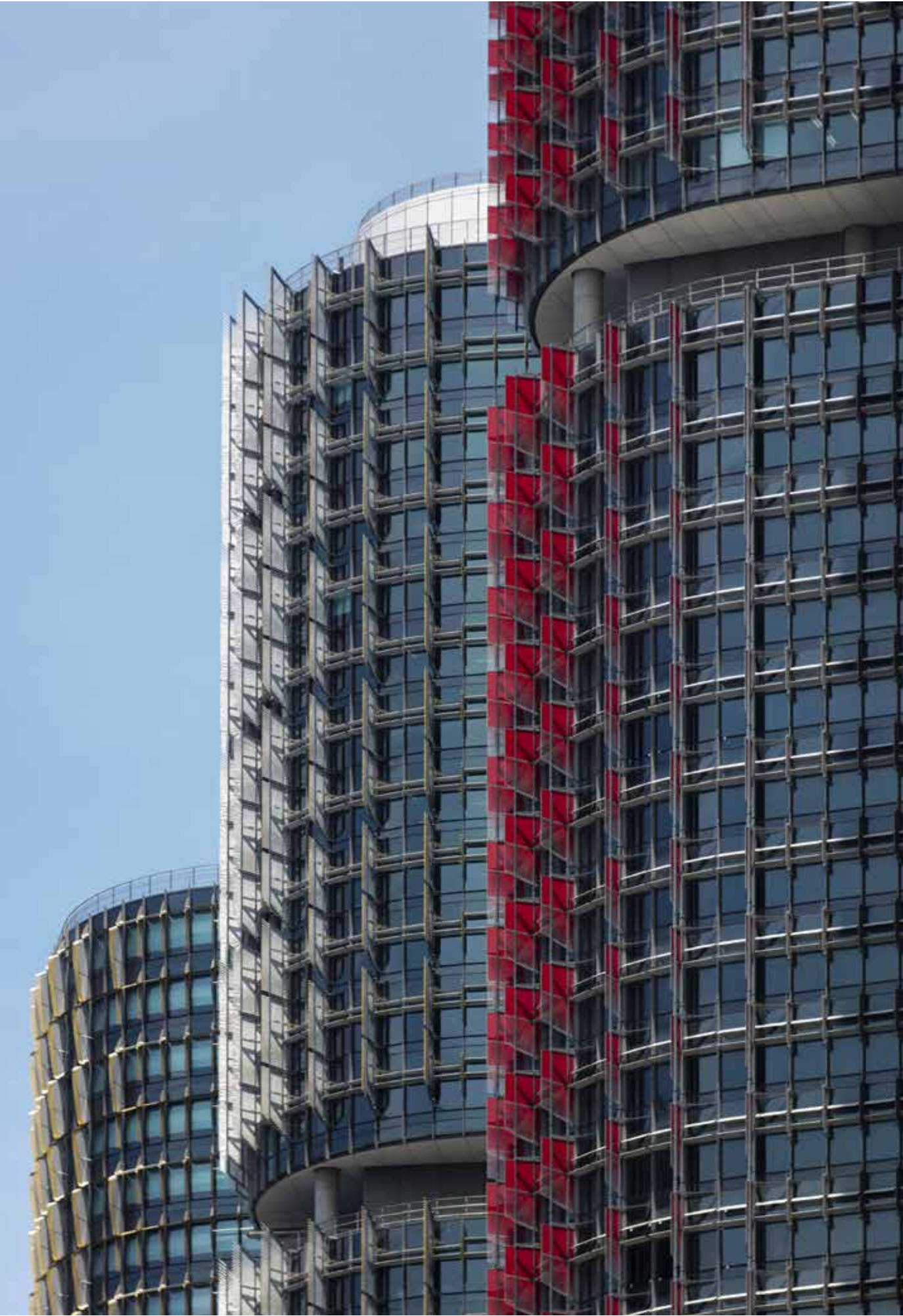
International Towers Sydney | The three towers viewed from Darling Harbour | Copyright holder © Brett Boardman Photography
