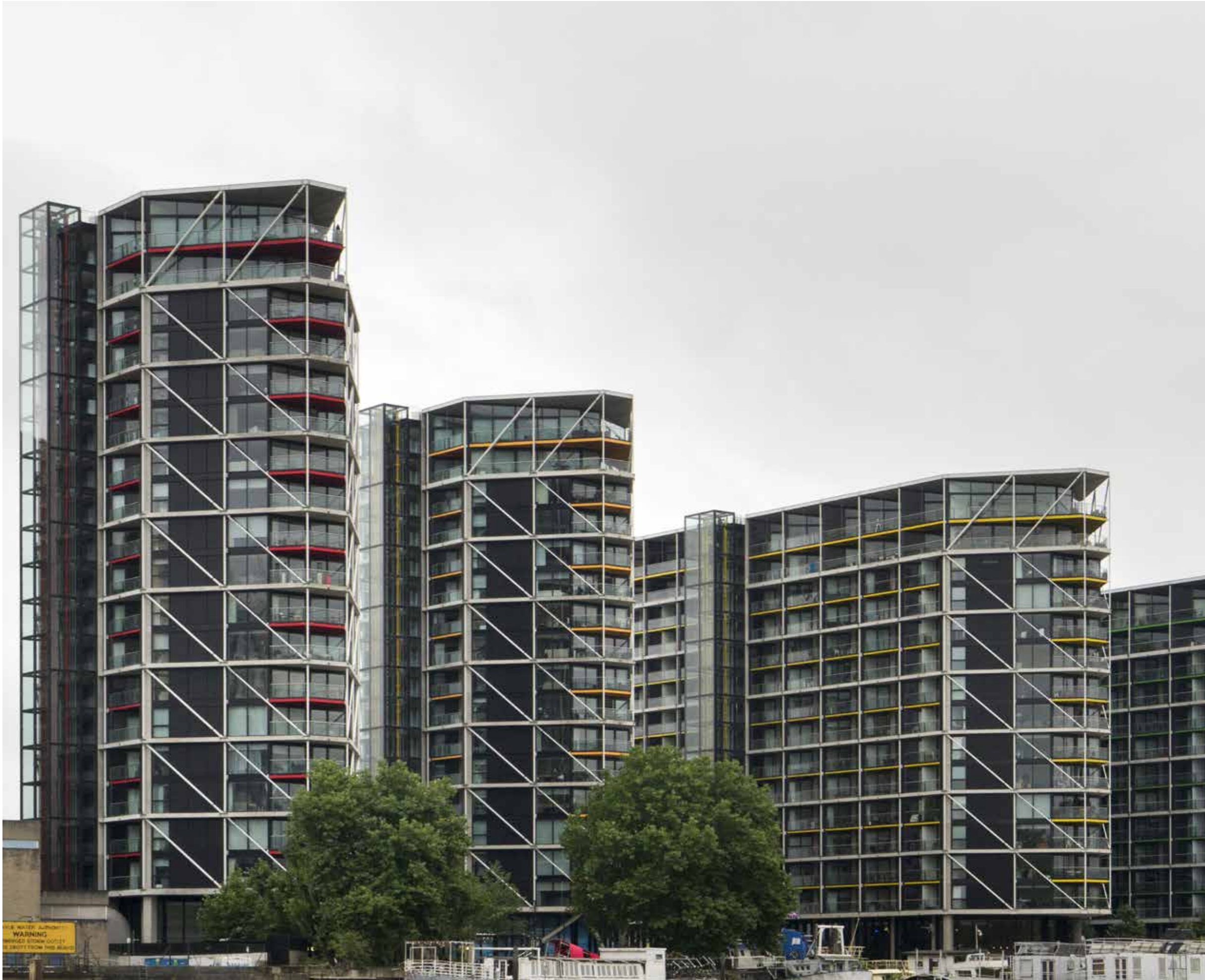
Anthony Coleman | Selected by Graham Stirk | The stepped forms of the buildings as seen from the River Thames
