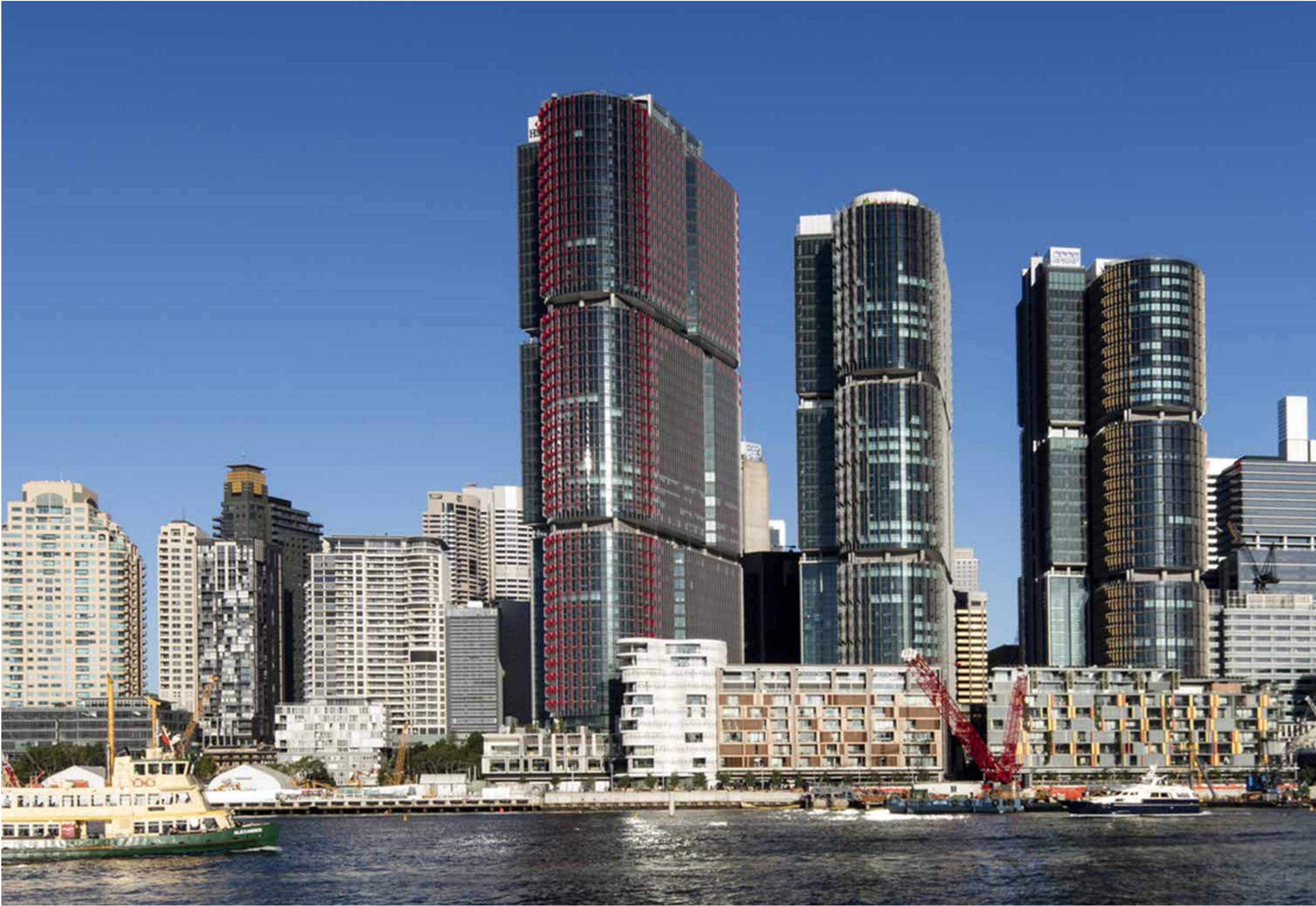
International Towers Sydney | The three towers viewed from Darling Harbour | Copyright holder © Brett Boardman Photography
