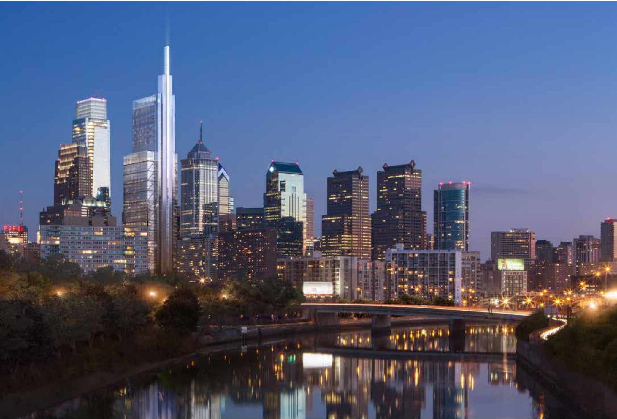
Comcast Innovation and Technology Centre dbox / Foster + Partners
