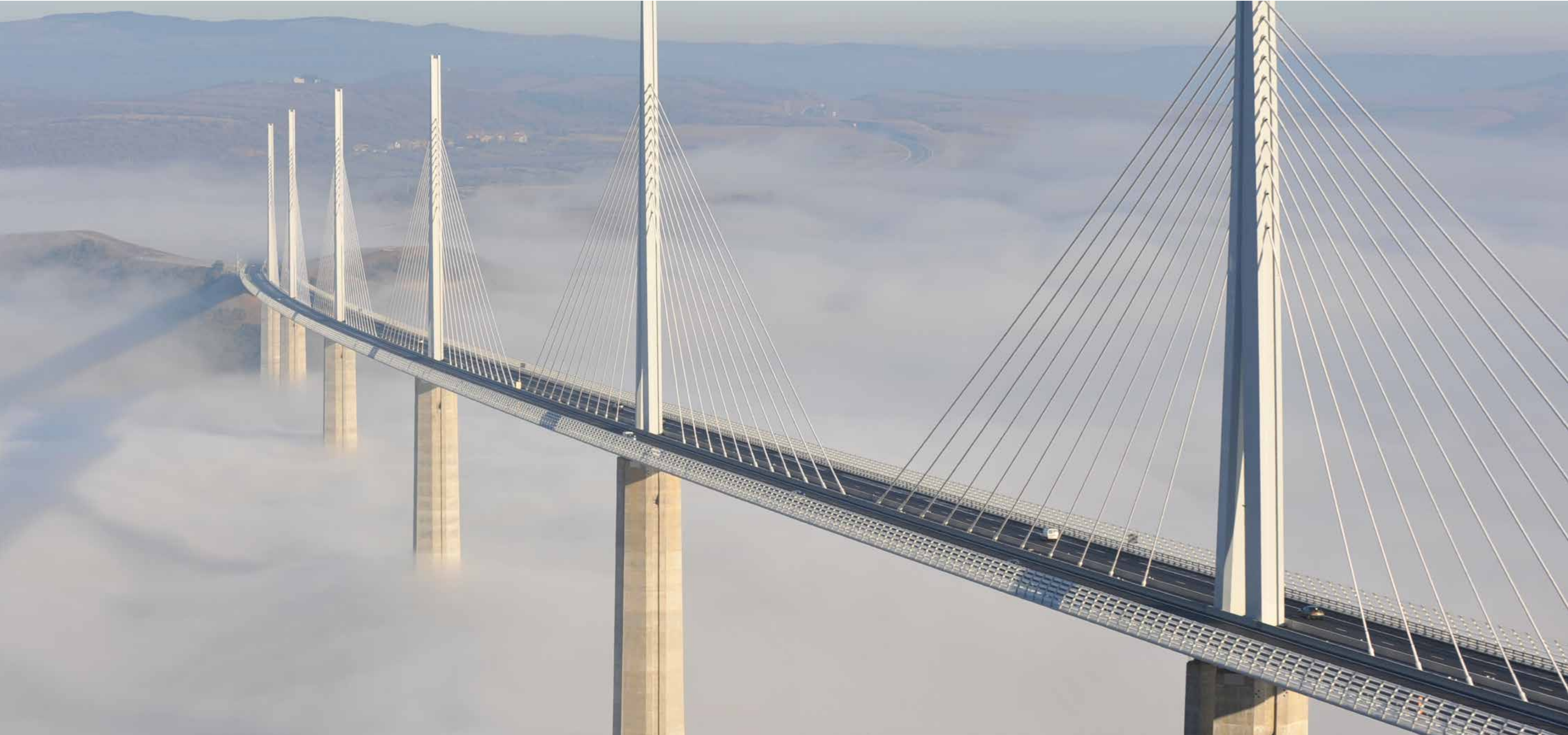
Millau Viaduct (main project number) Daniel Jamme/Eiffage
